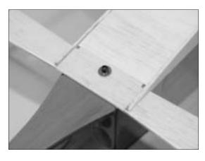
**Note**: The 4-40 socket head screw uses the 3/32" hex wrench.
